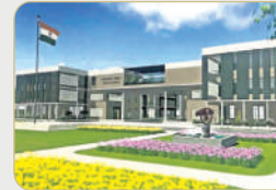
RR Dist. Collector Office - 25 Mins
